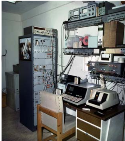
Control Room circa 1985
