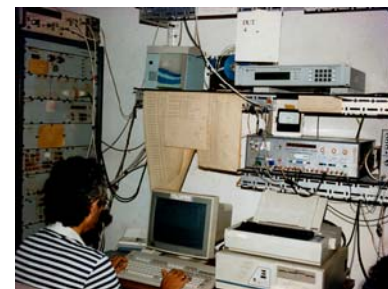
Control Room circa 1991
