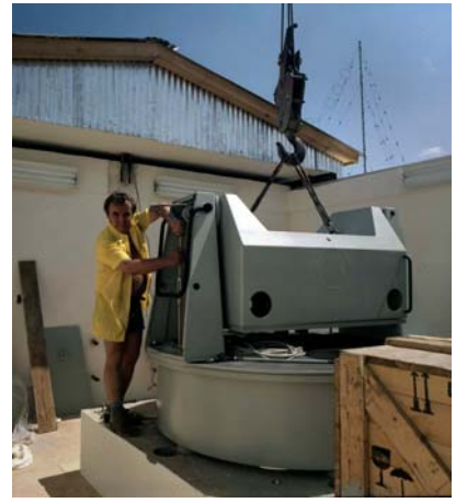
Assembly of the SBG system
